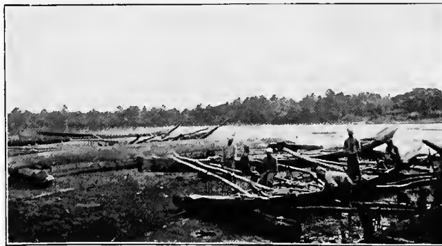
296. OPENING OUT THE BOAT-HULL.
